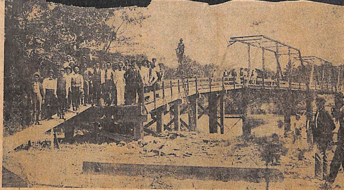
OLD LOVELACE BRIDGE , shown under construction shortly after the turn of the century. It connected Nos. 1 and 2 townships and was the result of faithful plugging by County Commissioner D. S. Lovelace who realized its necessity to make No. 1 township, south of the river, a real part of Cleveland county. This picture is the property of A. A. Alexander of Rt. 3, Union Rd., Gastonia, son of the
