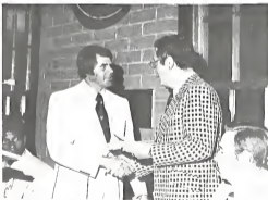
Ray DeHart, son of Mrs. Wayne DeHart and the late Mr. DeHart presents a check to Dr. Eugene Poizin in the amount of $61,859.10 at the Annual Building Sports Banquet. The check is to be applied to the construction of the new multi-purpose center. The basketball playing area will be named in memory of Mr. Wayne DeHart.
