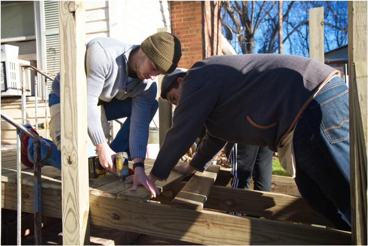
Students begin screwing in the support beams for the wheelchair ramp. Photo by: Mark Houser
